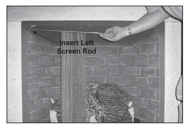
Figure 8.13 Insert Screen Rod
